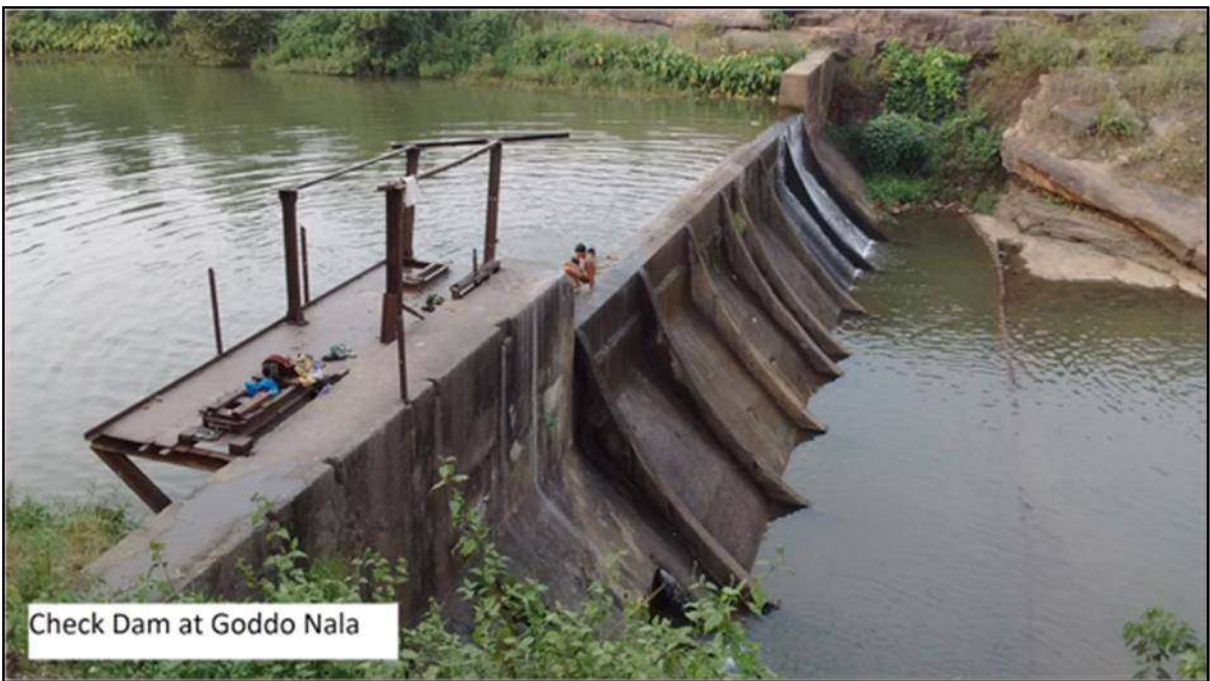
Fig: Check Dam near Godo Nallah
