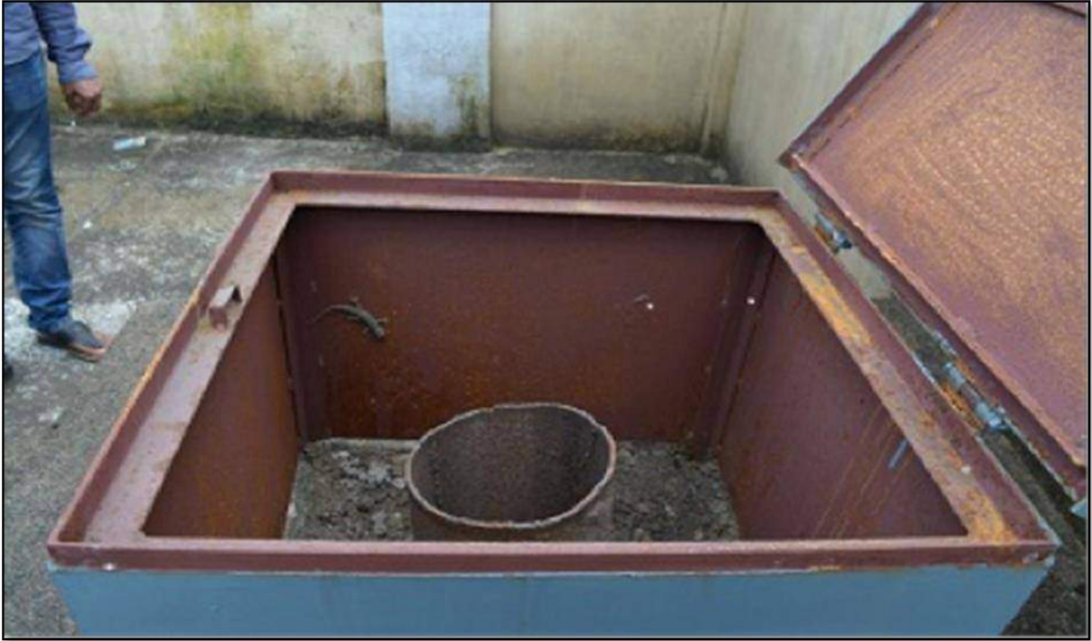
Fig: Piezometer Installed in Karo OCP
