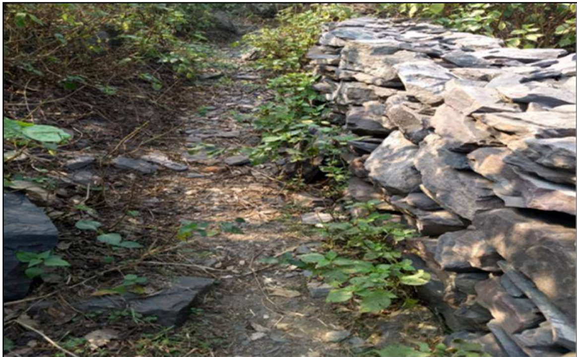
Fig: Garland Drain and Toe-wall
