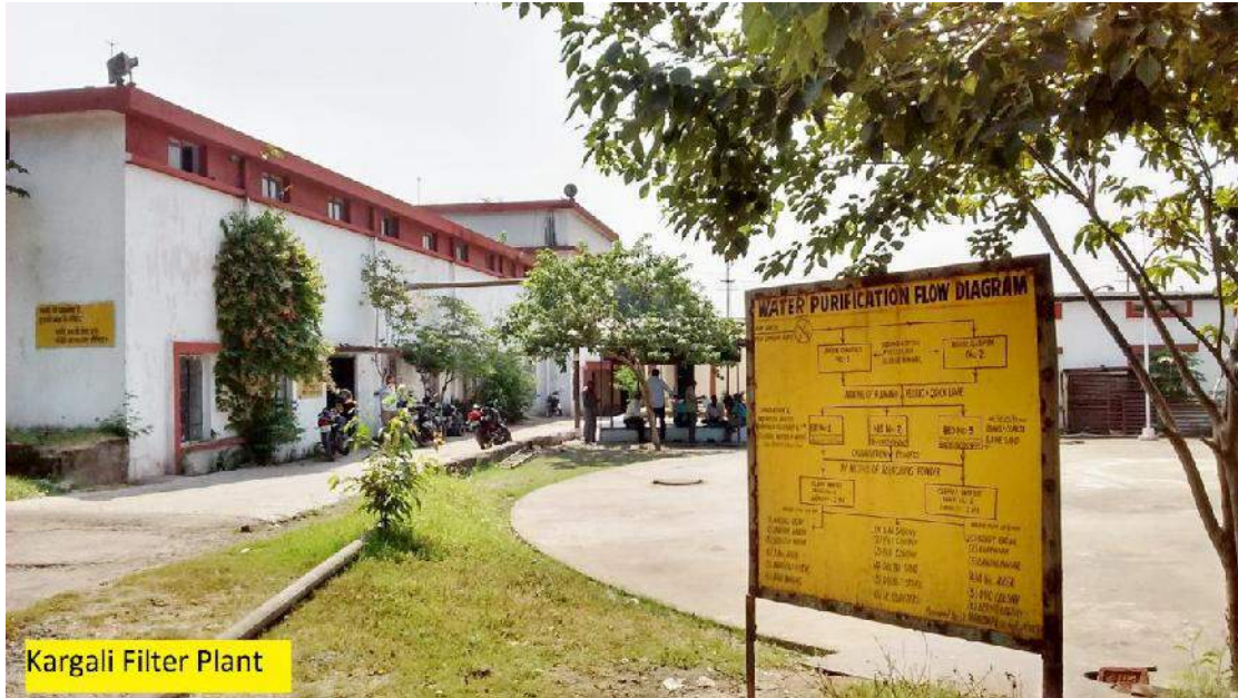
Figure-1: Water Filter Plant at B&K Area, CCL.
