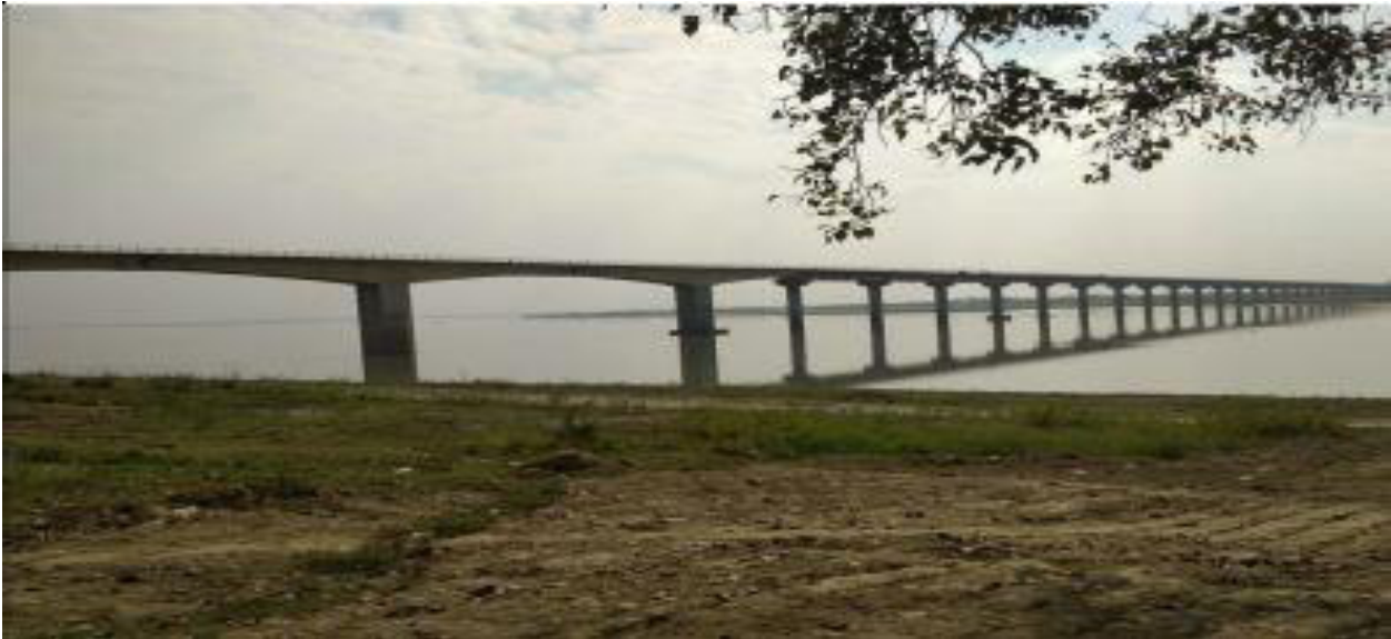
Photographs Showing the River Ghaghra at Km. 114+042
