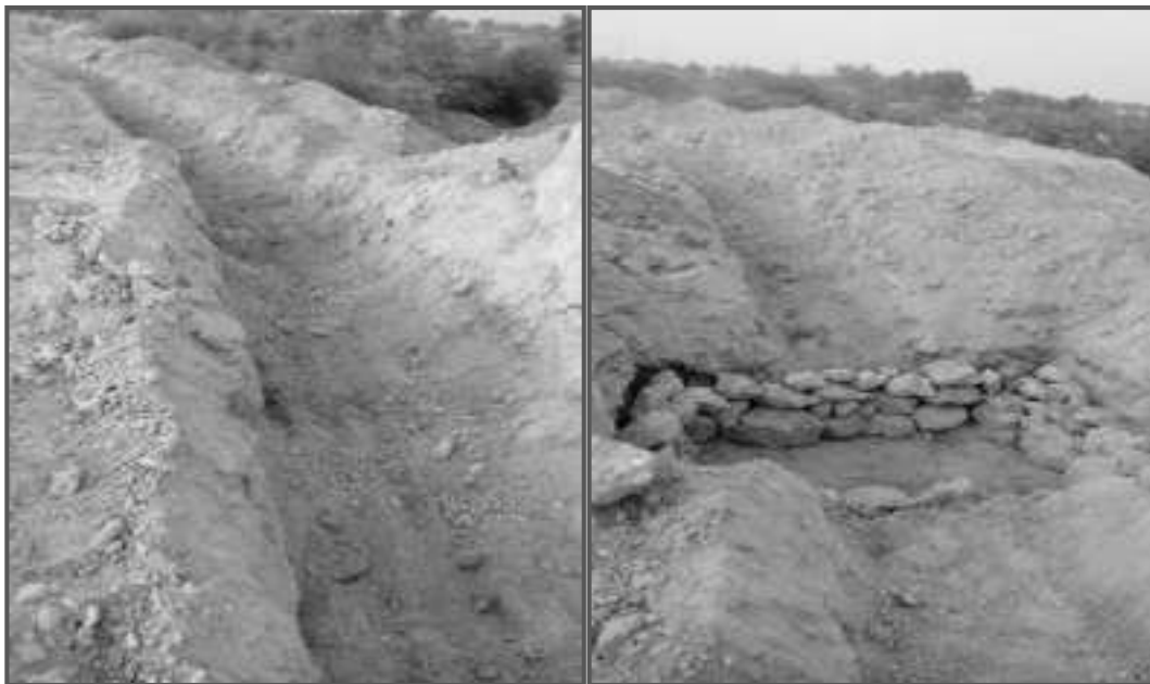
Photograph 13.3: Showing Garland Drains & Siltation Ponds
