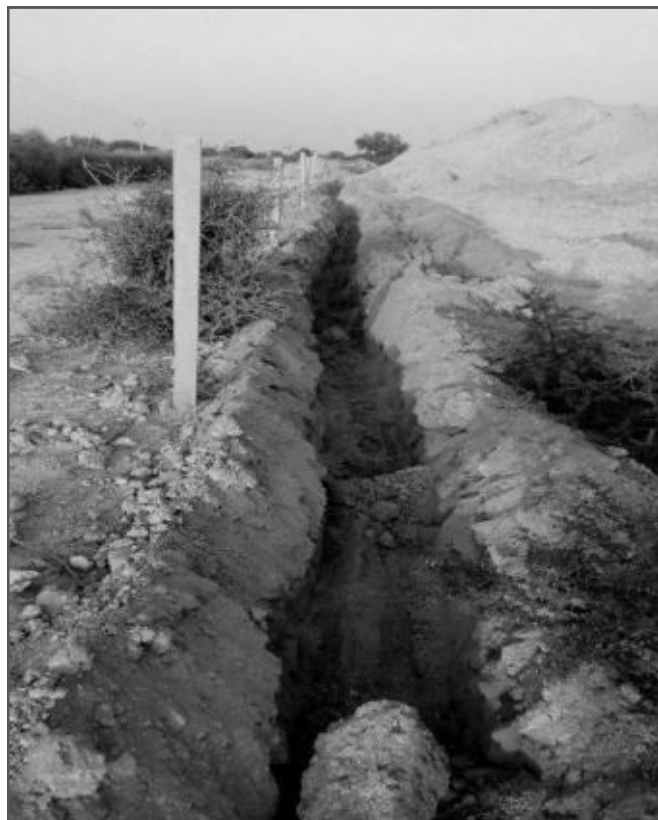
Photograph : Z- Showing Garland Drains and Siltation Pond.
