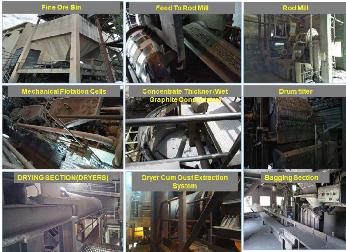
Figure 1-4 Beneficiation Plant Photographs
