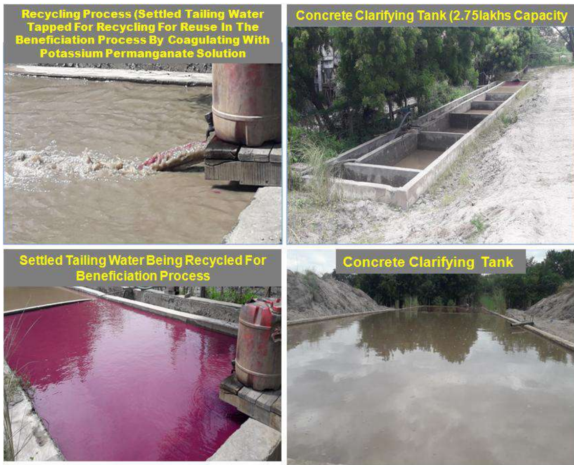
Figure 1-7Photographs of tailing water recycling
