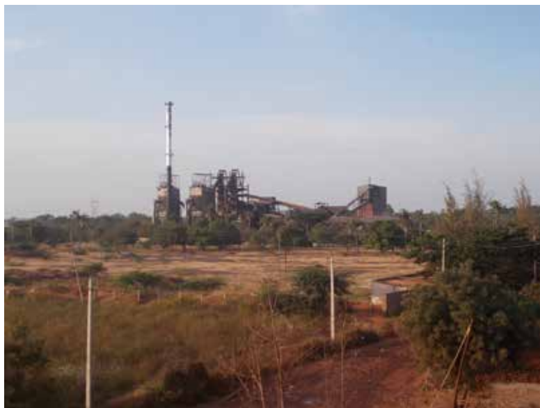
Photo 1.2: Sponge plant towards north side of the plant
