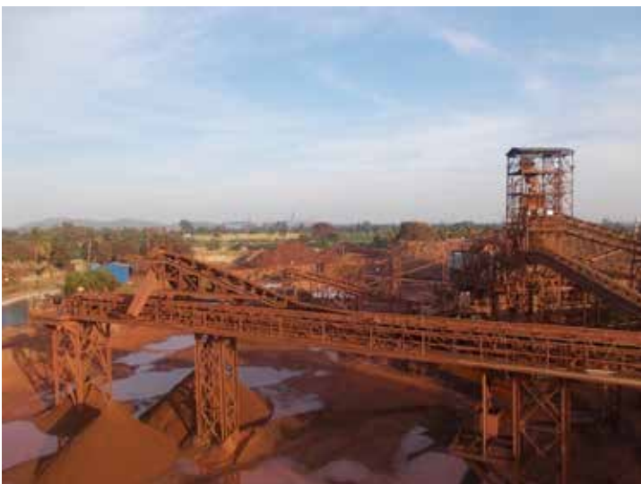
Photo 1.1: Photograph showing existing plant & machinery
