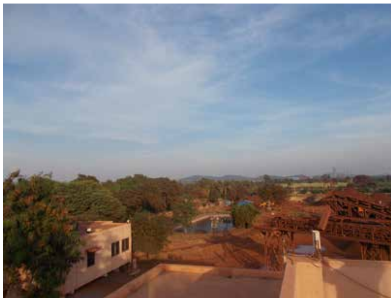
Photo 1.3: Towards eastern side of the plant
