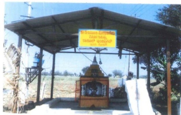
Roof for Anjuneya Temple at Hirebaganal Village
