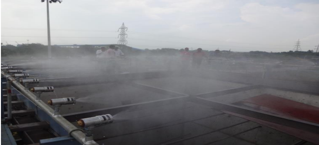
Fig. 21. Sprinkling water to suppress coal dust
