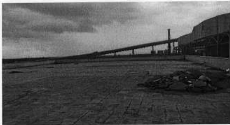
12. ESP Control Room
