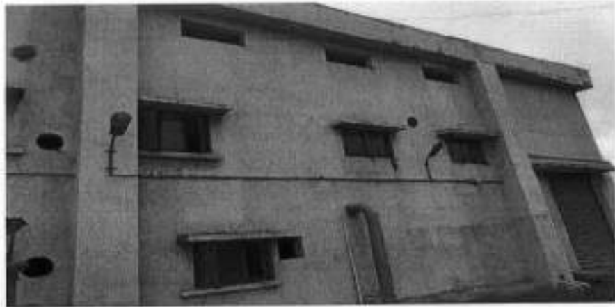
11. CT Pump House Terrace
