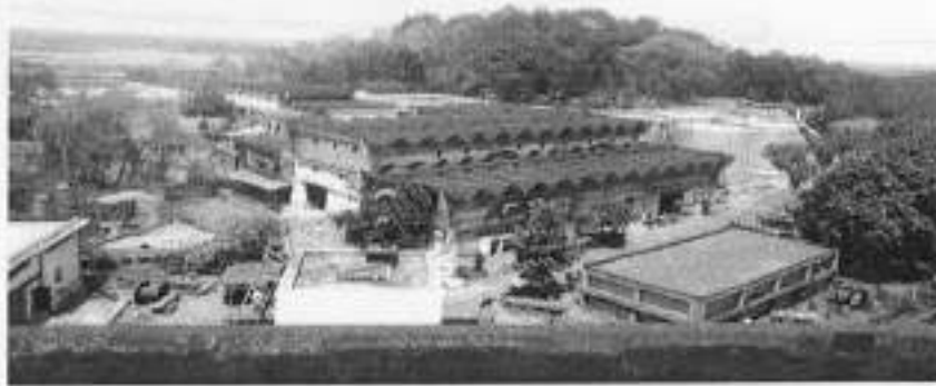
3. WTP -2 Building Terrace (Zigzag Top) A- 140 ft. x 130 ft. & B- 160 ft. x 80 ft.
