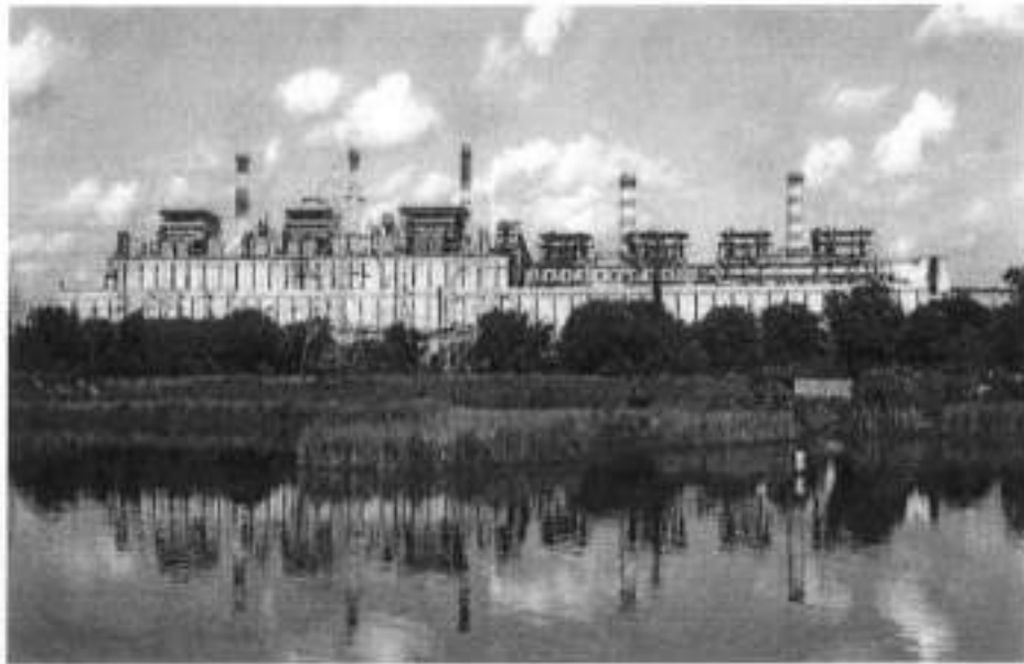
Koradi Thermal Power Station 210MW, Koradi, Nagpur
