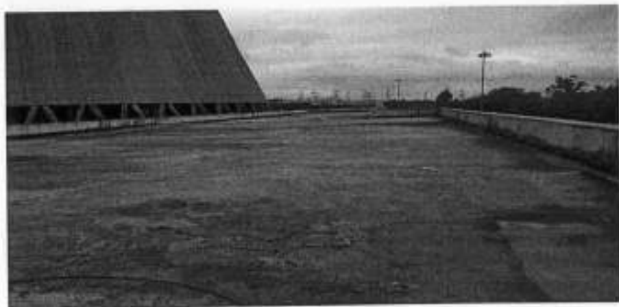
19. TTW & FW Pump House Terrace 300 ft. x 30 ft.
