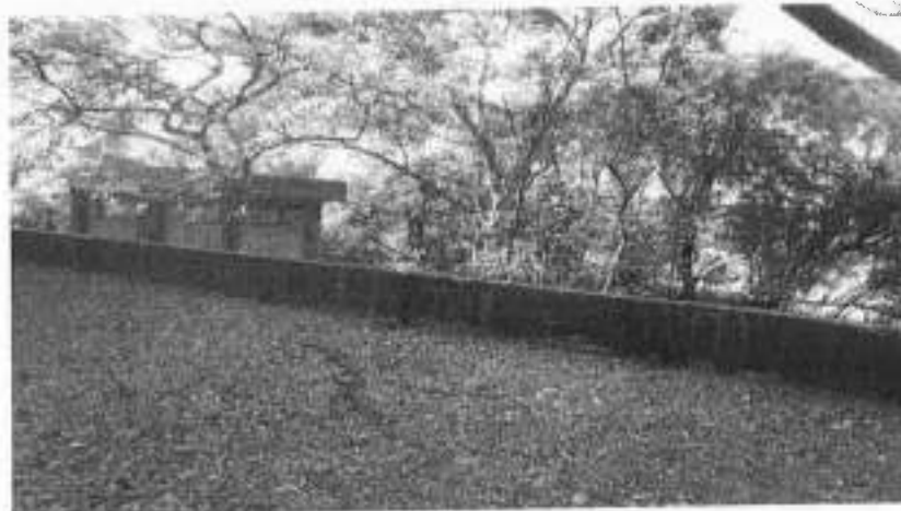
1. CTPL Building Terrace Down Portion 55ft. x 30 ft. (Shaded Area)
