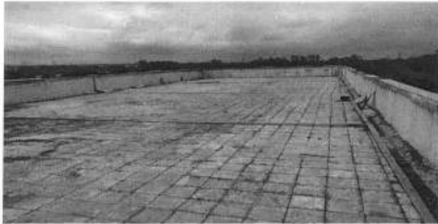
14. ACW Pump House Terrace 60 ft. x 30 ft.
