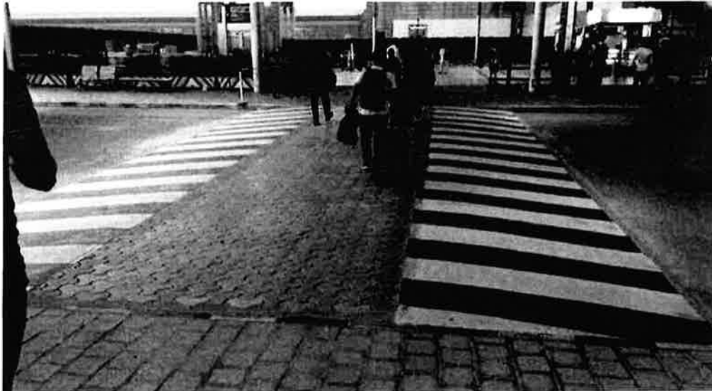
Plate: 5.2: Typical picture of High raised pedestrian crossing
