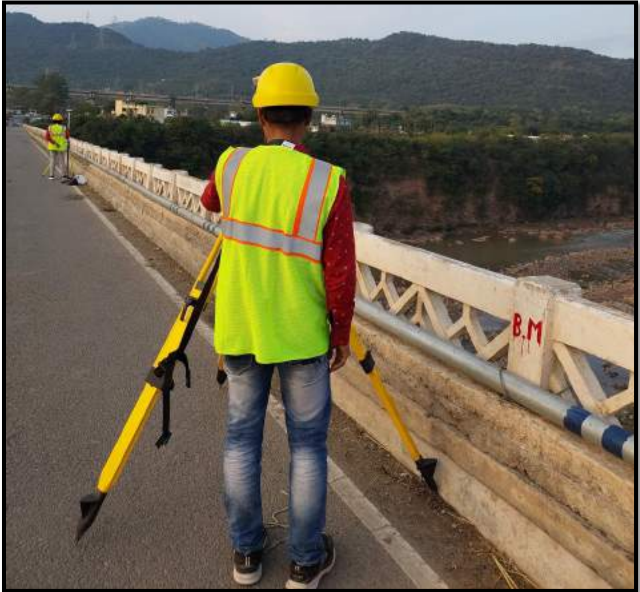
PHOTOGRAPH 9: Benchmark marked on Tawi River bridge in Jammu district.
