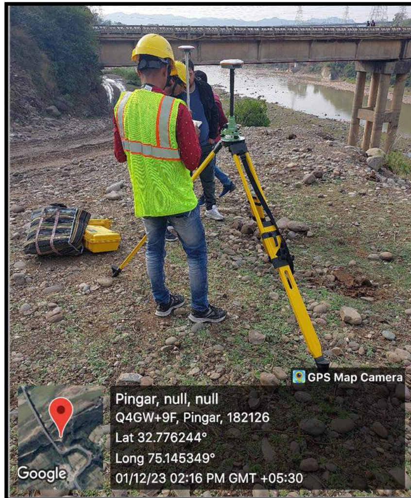
Picture of DGPS Survey in Sand / RBM zones.
