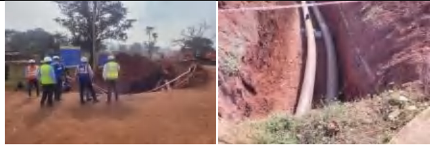
Lying of Slurry Pipeline (Stringing)
