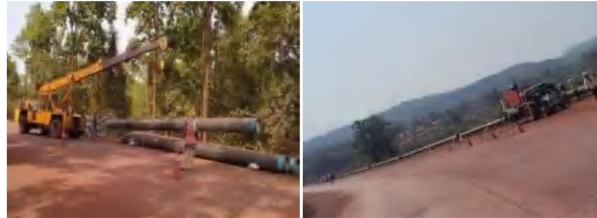
Lying of Slurry Pipeline (Stringing)
