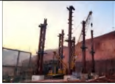
Feed Bin Building
