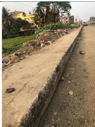
COVERED DRAINAGE SYSTEM (1200 MM WIDTH) INFRONT OF THE PROJECT SITE
