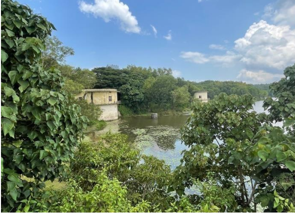
Anathazhachira at the lower end of the Park, with pumping stations
