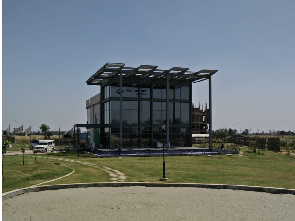
Photo – 1 (Front View of the site / sales office cum sample flat complex)
