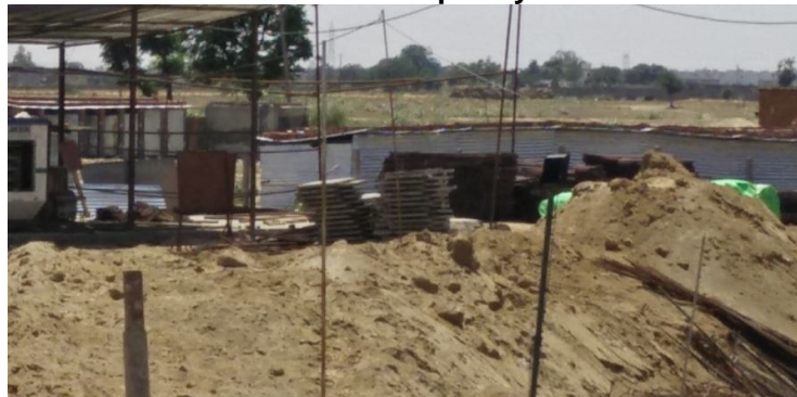
Photo – 11 (Pre-construction structures such as temporary site office and material store)
