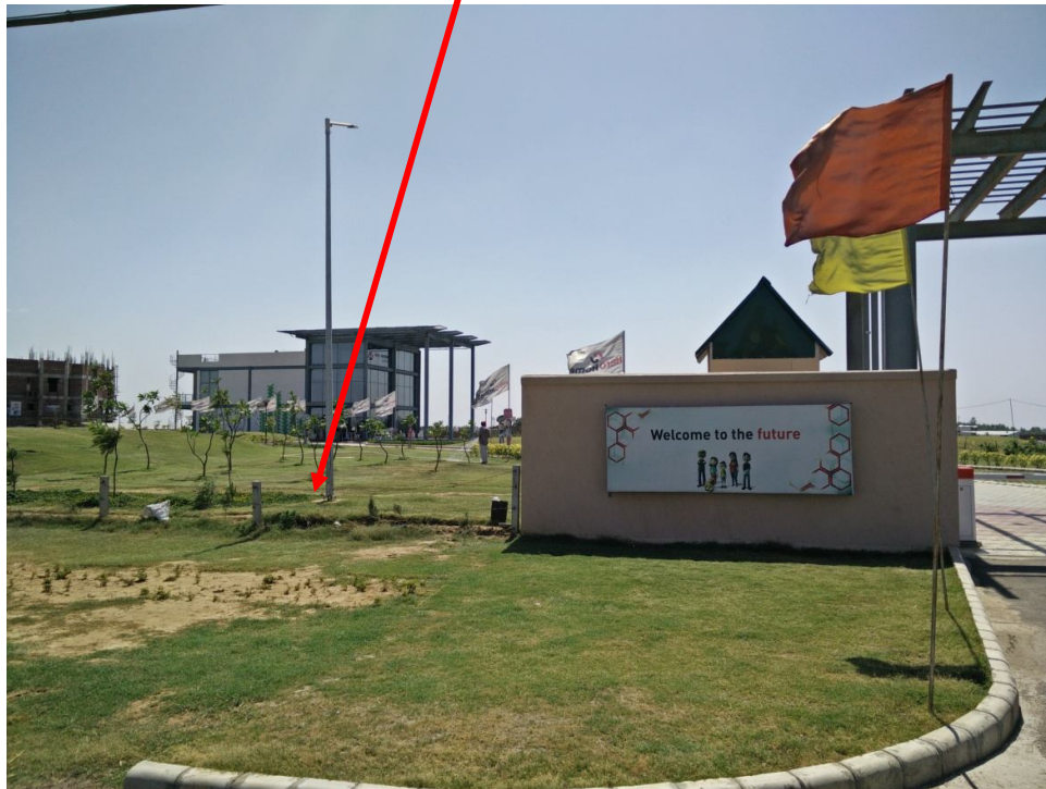
Photo – 6 (Wire Fencing)
