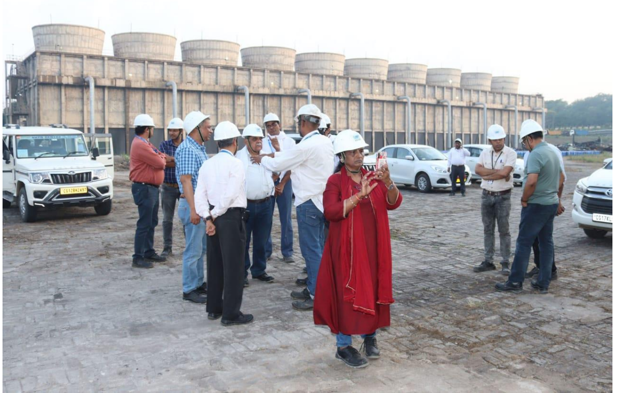
Figure 9: Induced Draft Cooling Towers at Korba STPP
