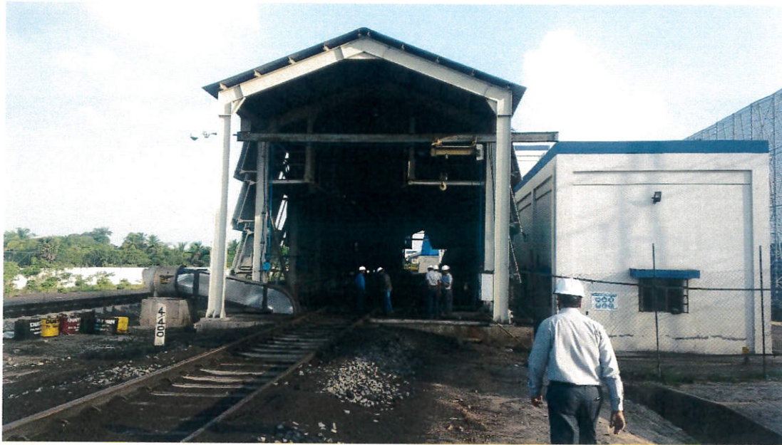
Figure 3. Coal unloading area (common to Phase 1 and 2)
