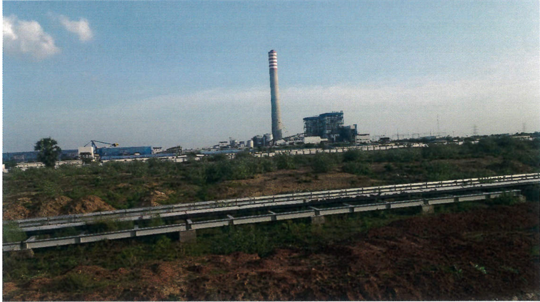
Figure 1. Panoramic view of Phase 1 plant from behind land earmarked for Phase 2
