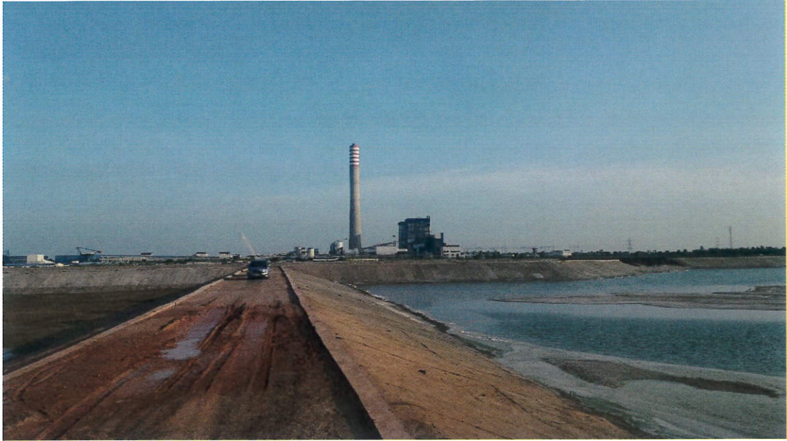
Figure 5. View of both ash ponds common to both phases (only one in use)
