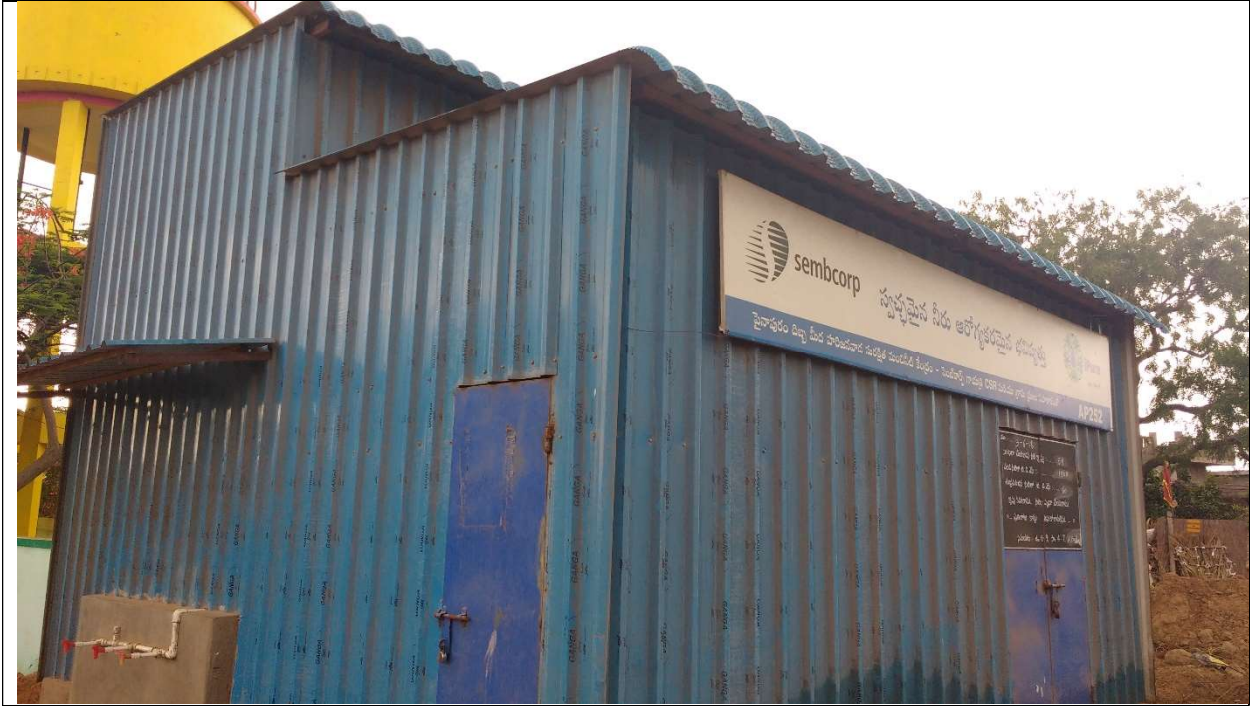
3. RO treatment plan provided in Pinapuram Village by M/s Sembcorp Gayatri Power Ltd.
