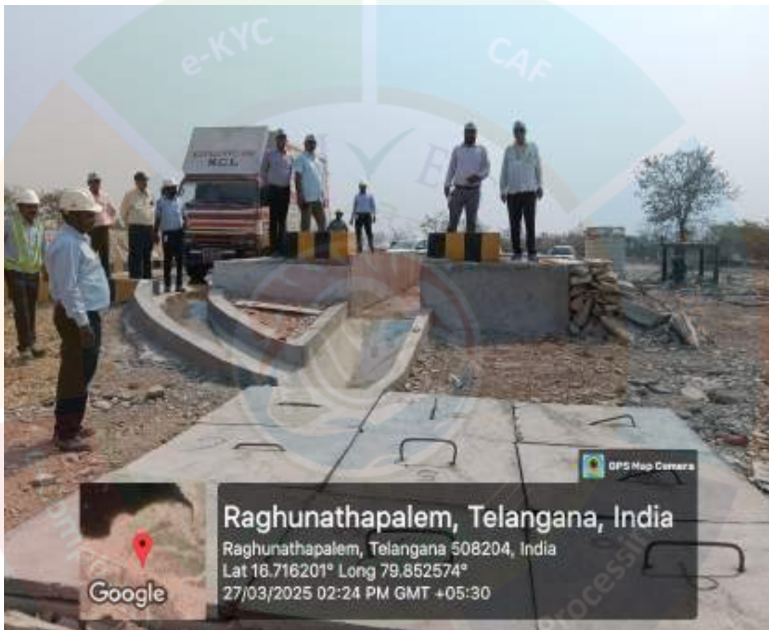
Oil and Grease Trap without shade
