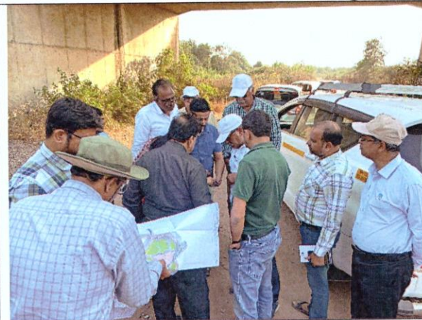
Ch 2+150 Vashi-Panvel railway underpass.
