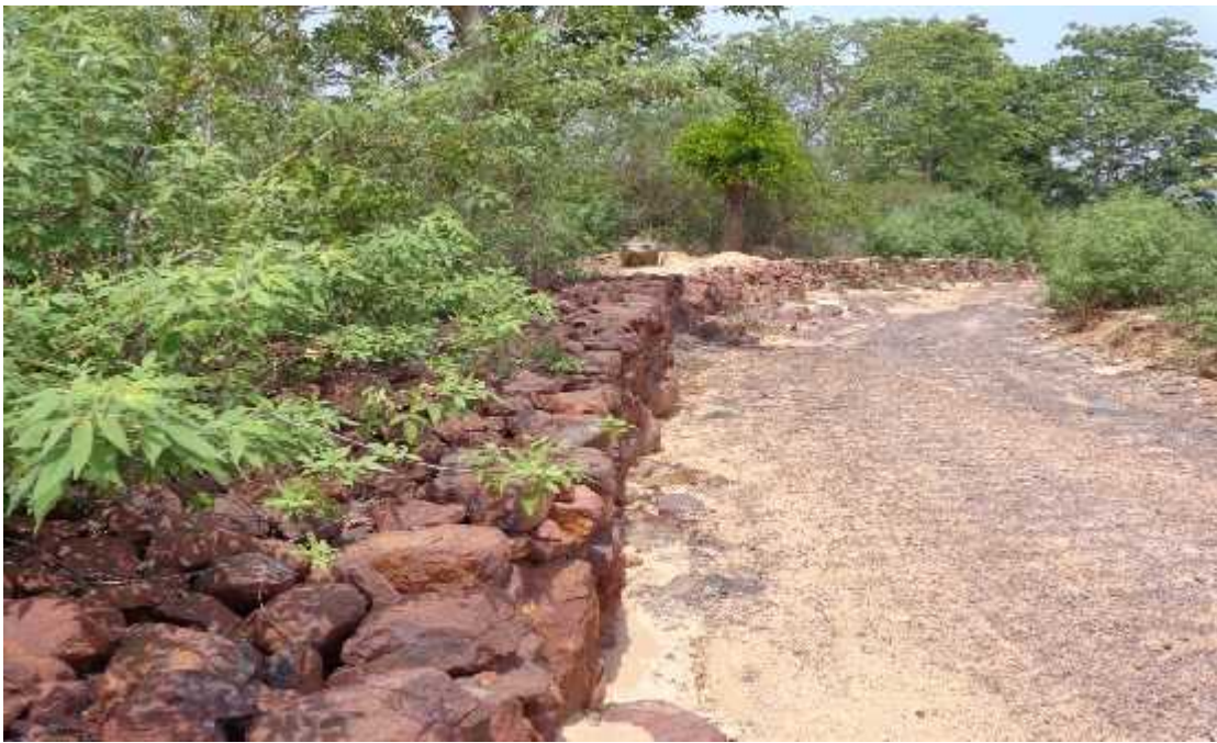
STONE WALL ALONG THE BANK OF SEASONAL NALLA
