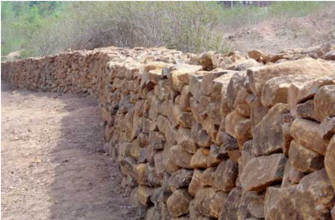
BOULDER WALL ON SEASONAL NALA
