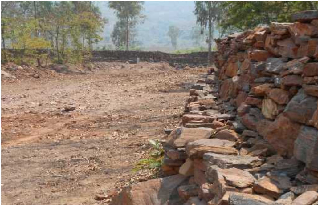
BOULDER WALL ON SEASONAL NALA
