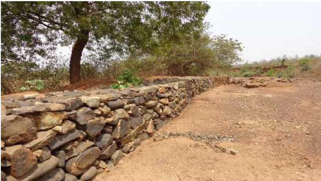
BOULDER WALL AT VILLAGE BALIKHANI
