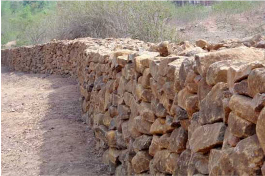
BOULDER WALL NEAR VILLAGE SUNDHAL
