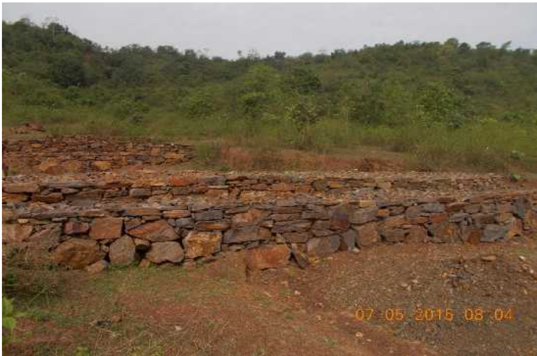
STONE WALL AT SEASONAL NALLA
