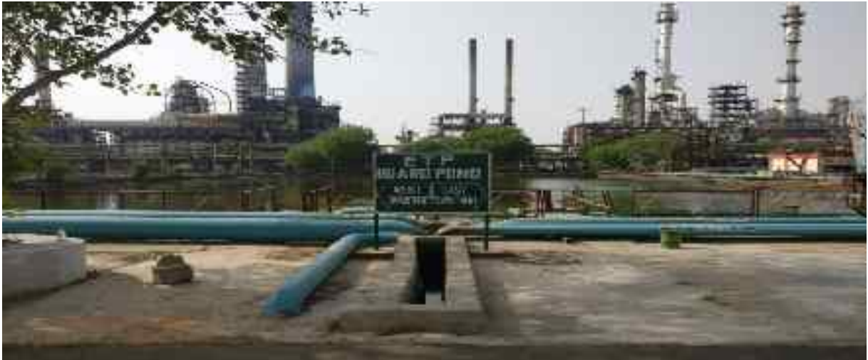
Figure 2-4 Photographs of Effluent Treatment Plant
