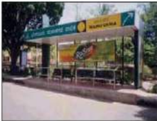
Well-maintained Bus Stop
