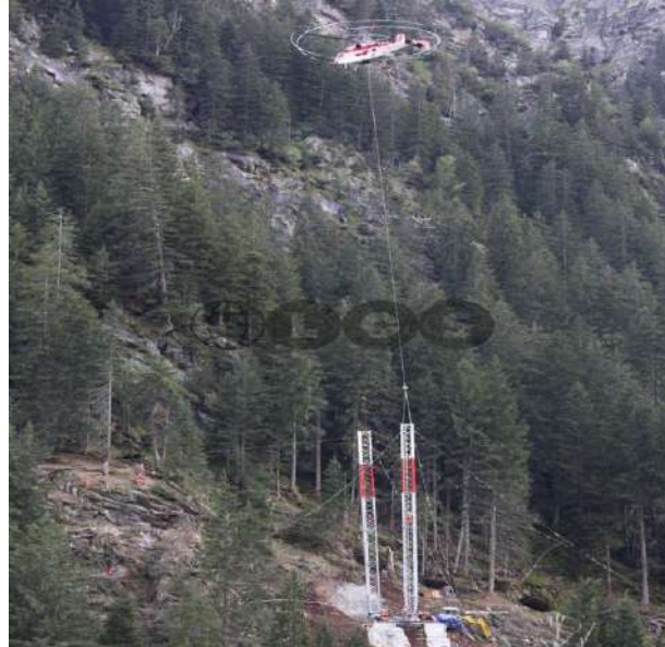
Figure 7.14 : Use of Helicopter for tower erecting job –Risky work
