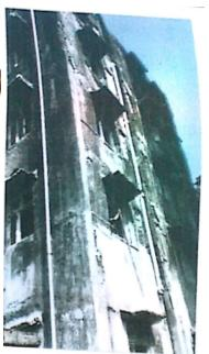
Since RCC structure of G+4 upper floors were extremely dilapidated and beyond repair the same was decided by MCGM to demolish and reconstruction of the same building on the same plinth area with some modified requirement s of Health post and dispensary are now proposed.
