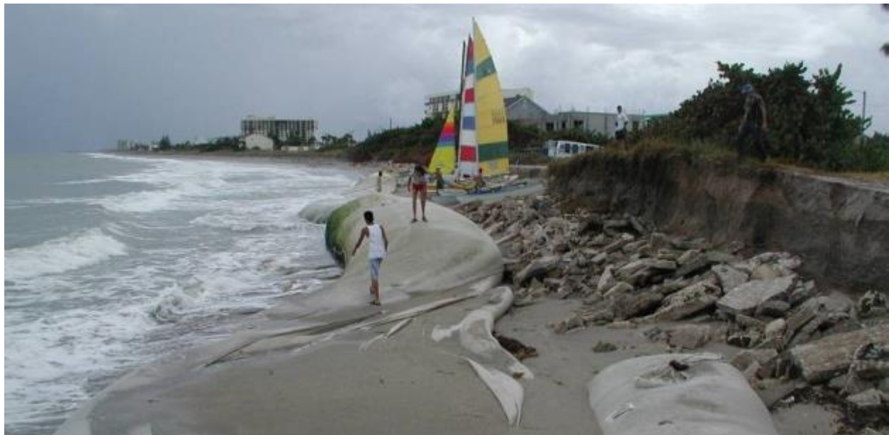
Figure 3.28 Impacts due to wave reflection: toe scour, undermining, differential settlement
