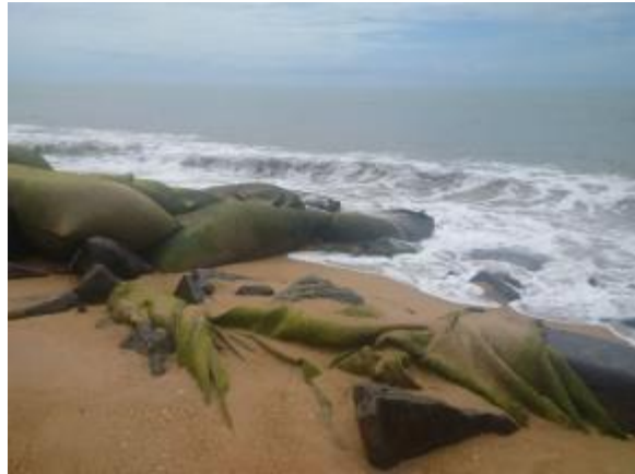
Figure 3.30 Dislodged and damaged containers, Ullal, Karnataka
