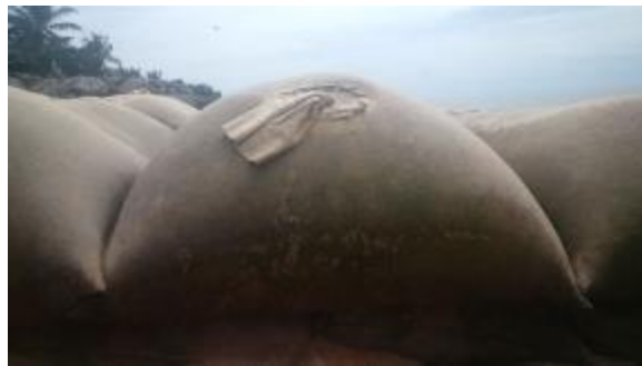
Figure 3.33 Effective closure of fill ports is critical to the long-term integrity of the structure, as experience had shown that ports, which allow the loss of fill material results in deflation of the containers.
