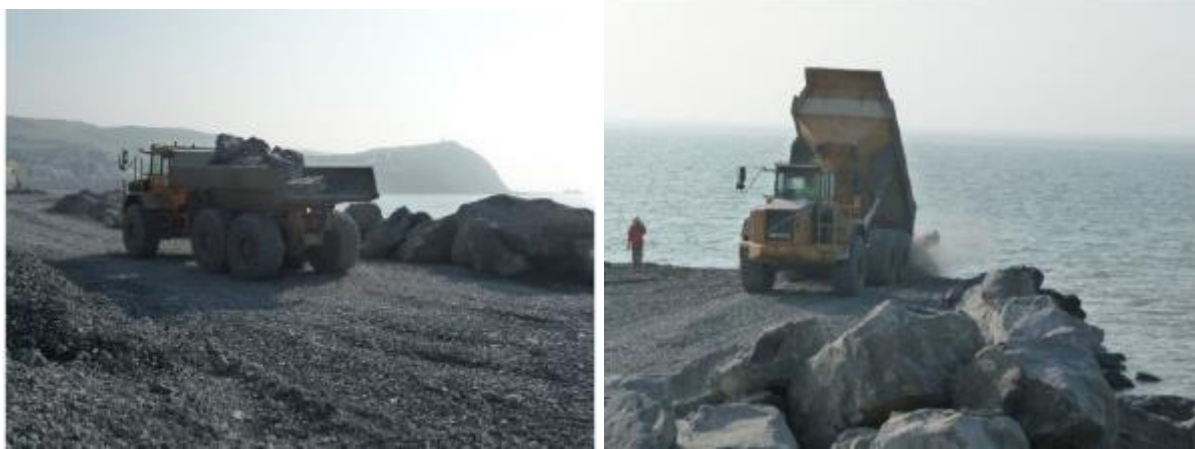
Figure 3.14. Dump truck transporting armour stone to construction site
