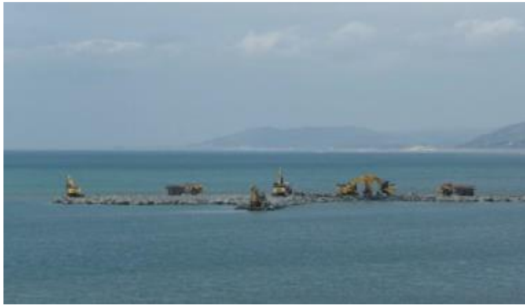
Figure 3.17 Reef construction underway and dumper trucks delivering armour stones
