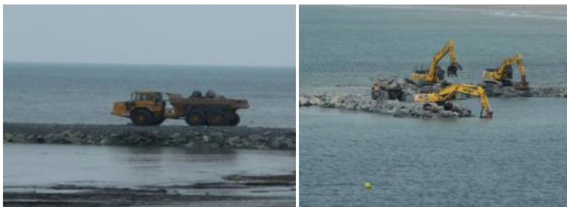
Figure 3.15 Dumper truck carrying armour stone to the seaward end of the reef over a purpose built causeway and placement of armour rocks from the causeway using excavators
