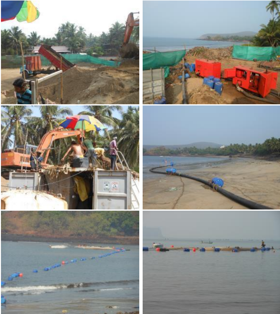
Figure 3.27. Mirya reef construction: land based sand slurry pumping
