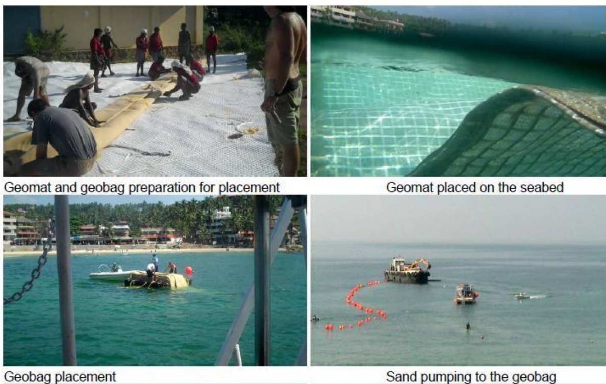
Figure3.26. Geotextile megacontainer pre-deployment preparations ,placement and underwater filling
