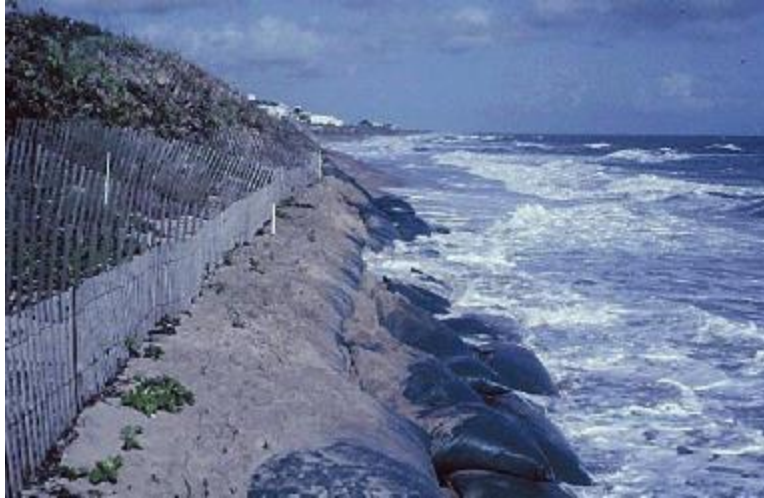
Figure 3.29 Failure due to Undermining Most common failure mode
