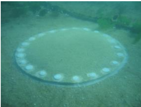
Figure 3.33 Effective closure of fill ports is critical to the long-term integrity of the structure, as experience had shown that ports, which allow the loss of fill material results in deflation of the containers.
