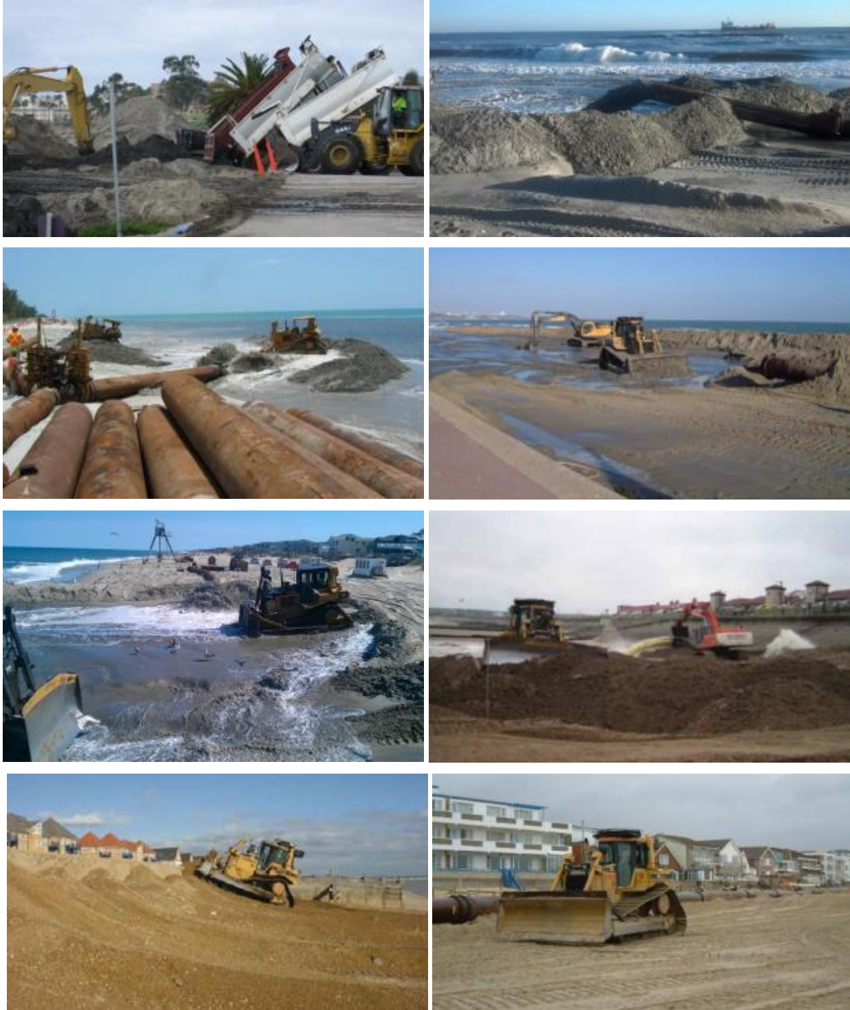
Fig 3.36 Photographs showing various activities involved in beach nourishment works
