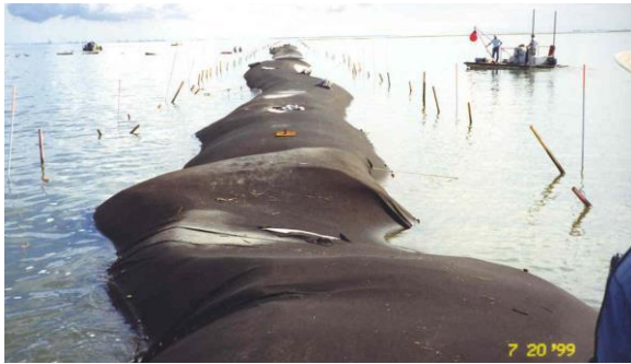
Figure 3.32 Under-filling could cause sand movement inside the containers under wave action and over-filling could affect the seam efficiency
