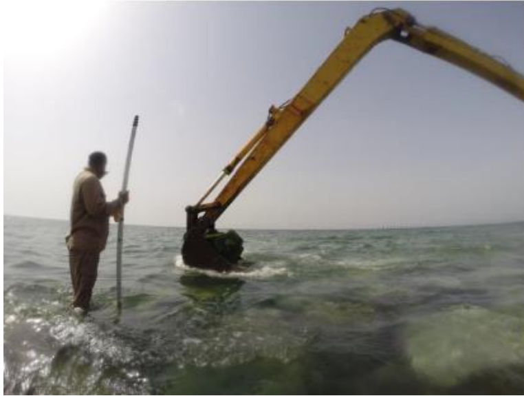
Figure 3.18 Placing 3-6t armour rock tightly at low tide (UAE project picture)
