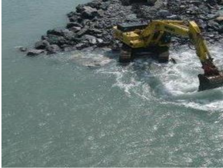
Figure 3.16 Excavator placing the armour stone upwards from the sea bed
