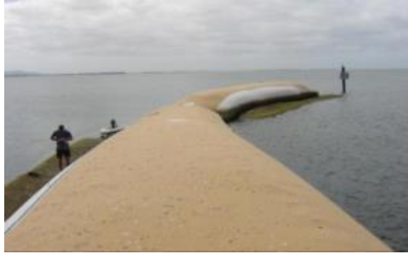
Figure 3.32 Under-filling could cause sand movement inside the containers under wave action and over-filling could affect the seam efficiency
