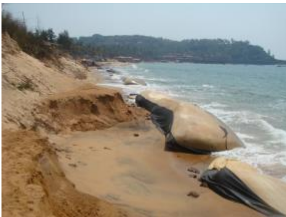
Figure 3.31 Punctured woven geotextile - Candolim, Goa
