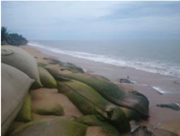
Figure 3.30 Dislodged and damaged containers, Ullal, Karnataka
