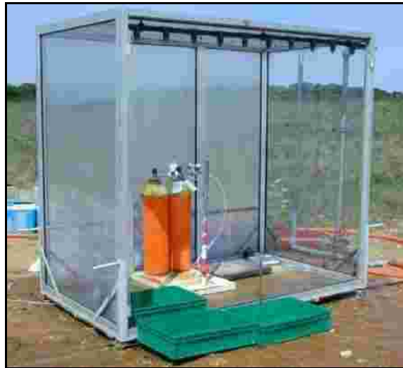
Figure 7.2 Shed for Chlorine Tonner
