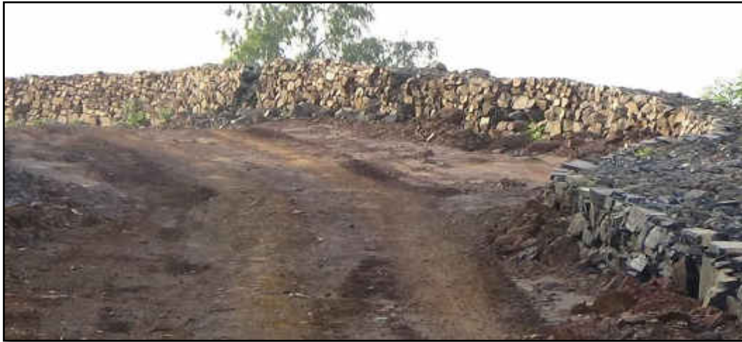
26 Meters New Stone Wall has been constructed Along the Haul Raod Side to Prevent Soil Erosion
