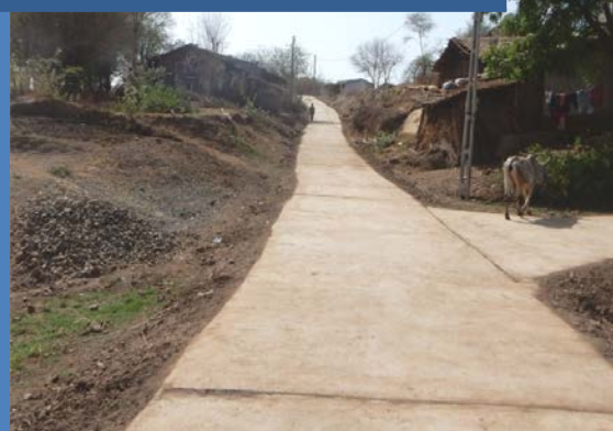
CC Road, Timberwa village
