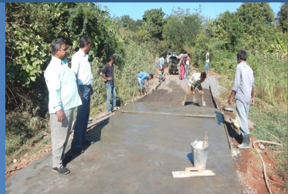
Site engineer with Sarpanch during construction phase
