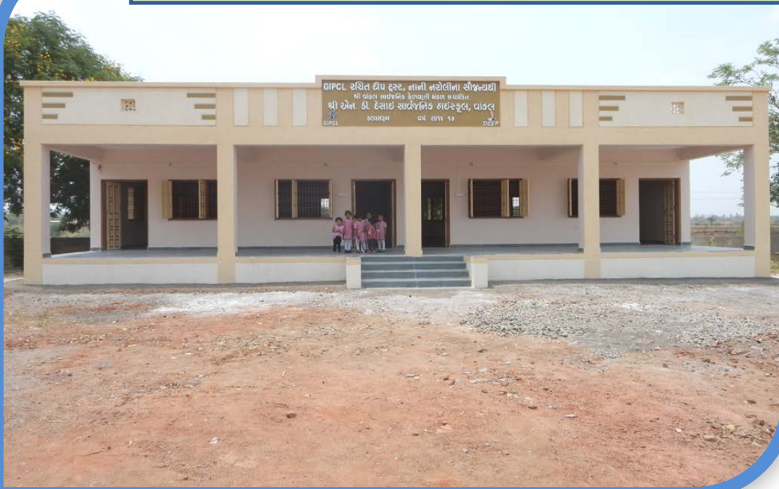
The newly constructed class room at Vankal High School
