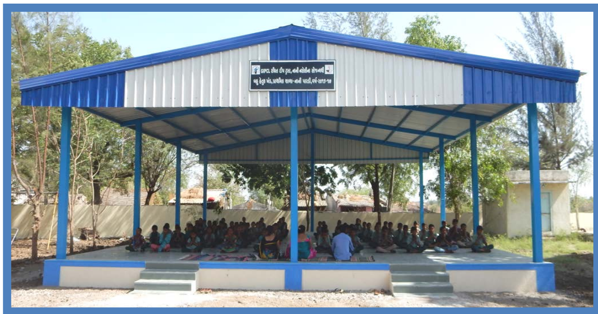
The Multipurpose Shed at Government Primary School, Nani Pardi
