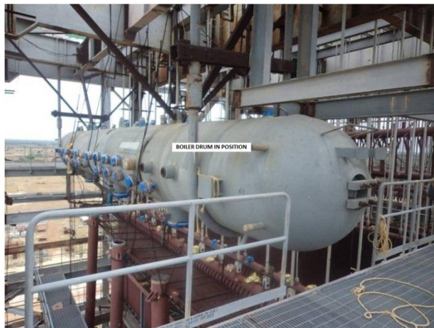
BOILER DRUM IN POSITION
