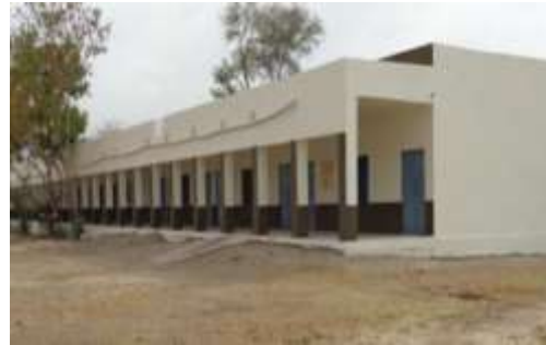
Renovation of Sr. Sec.. School Kotri
