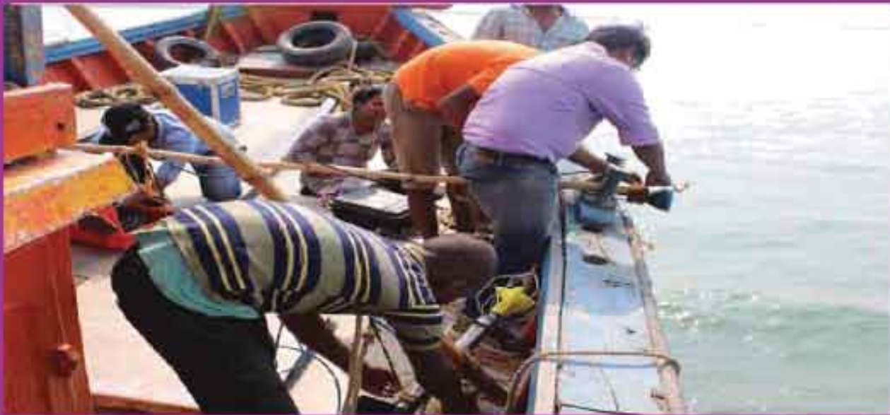
P17: Mounting of ADCP and Eco-Sounder for Bathymetry Survey at Proposed Water Intake Site of GTPP
