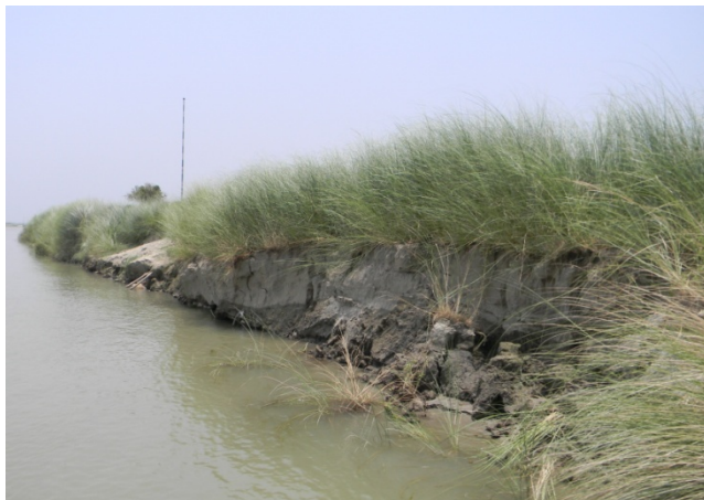
Fig. 51. Dense infestation of grass unable to prevent river bank erosion near Nabadwip
