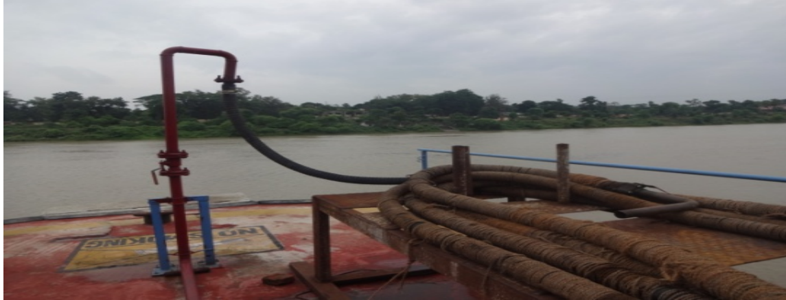
Fig. 6. Bunkering arrangements at Farakka
