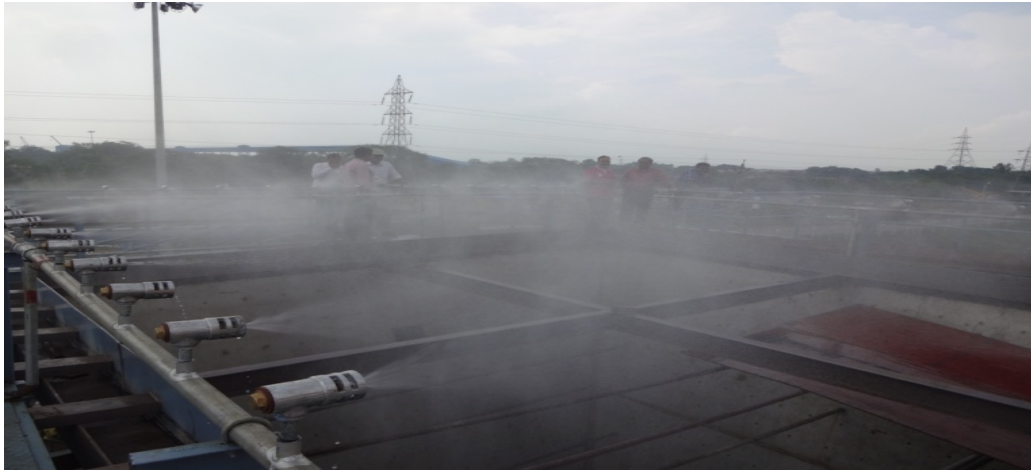
Fig. 10. Sprinkling water to suppress coal dust
