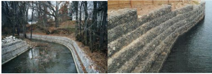
Fig. 118. Concrete walls and gabions
