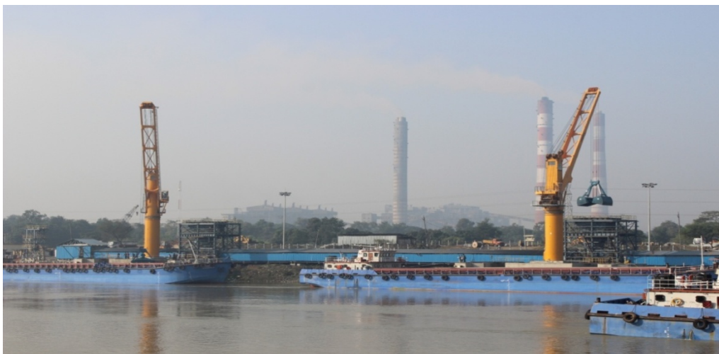
Fig. 7. Coal unloading point at Farakka
