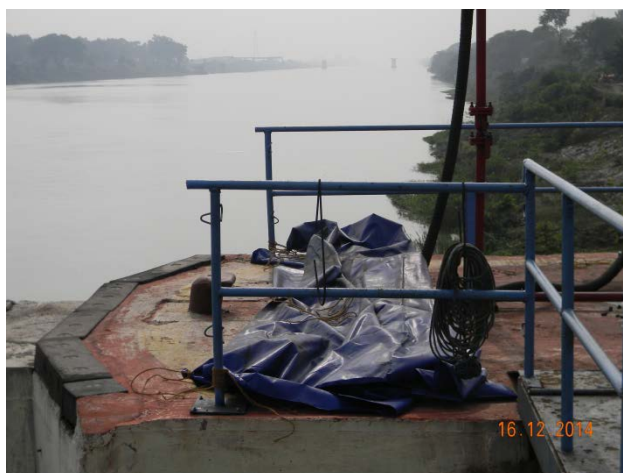
Fig. 47. Tarpaulin sheet used to prevent coal particle scattering into the river
