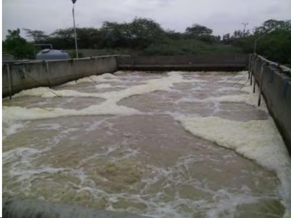
ETP – Equalization Tank
