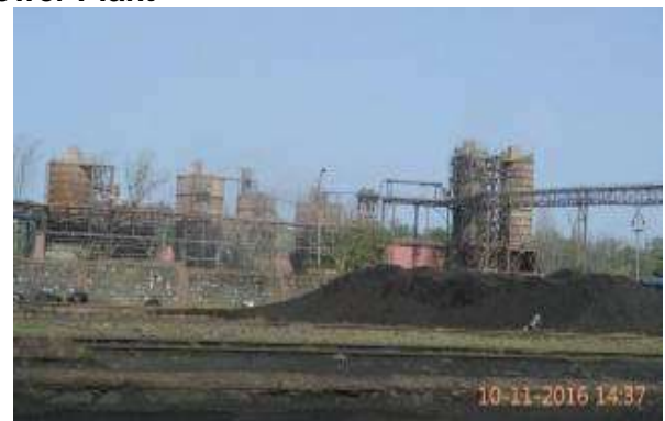
Fly ash Silos
