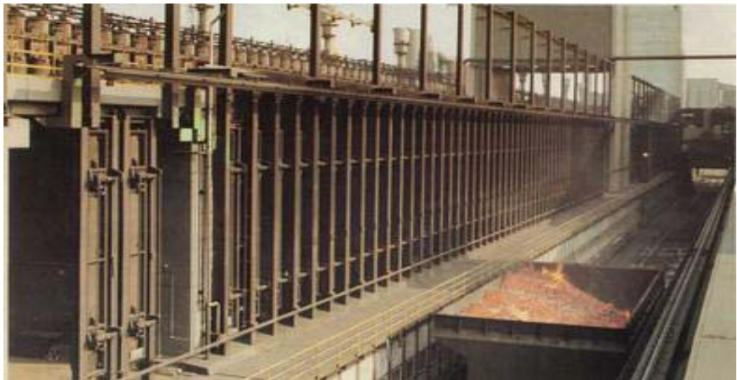
Figure 3-3: Coke Side of a By-Product Coke Oven Battery
