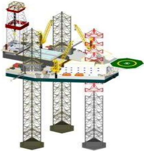
Figure 7:A Typical View of Jack-up Rig
