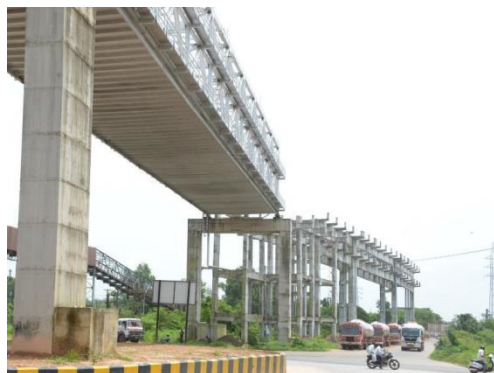
MSEZL Elevated Pipe Rack NH Crossing
