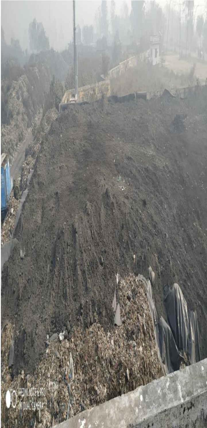
Existing Landfill Site ( View – 1 )
