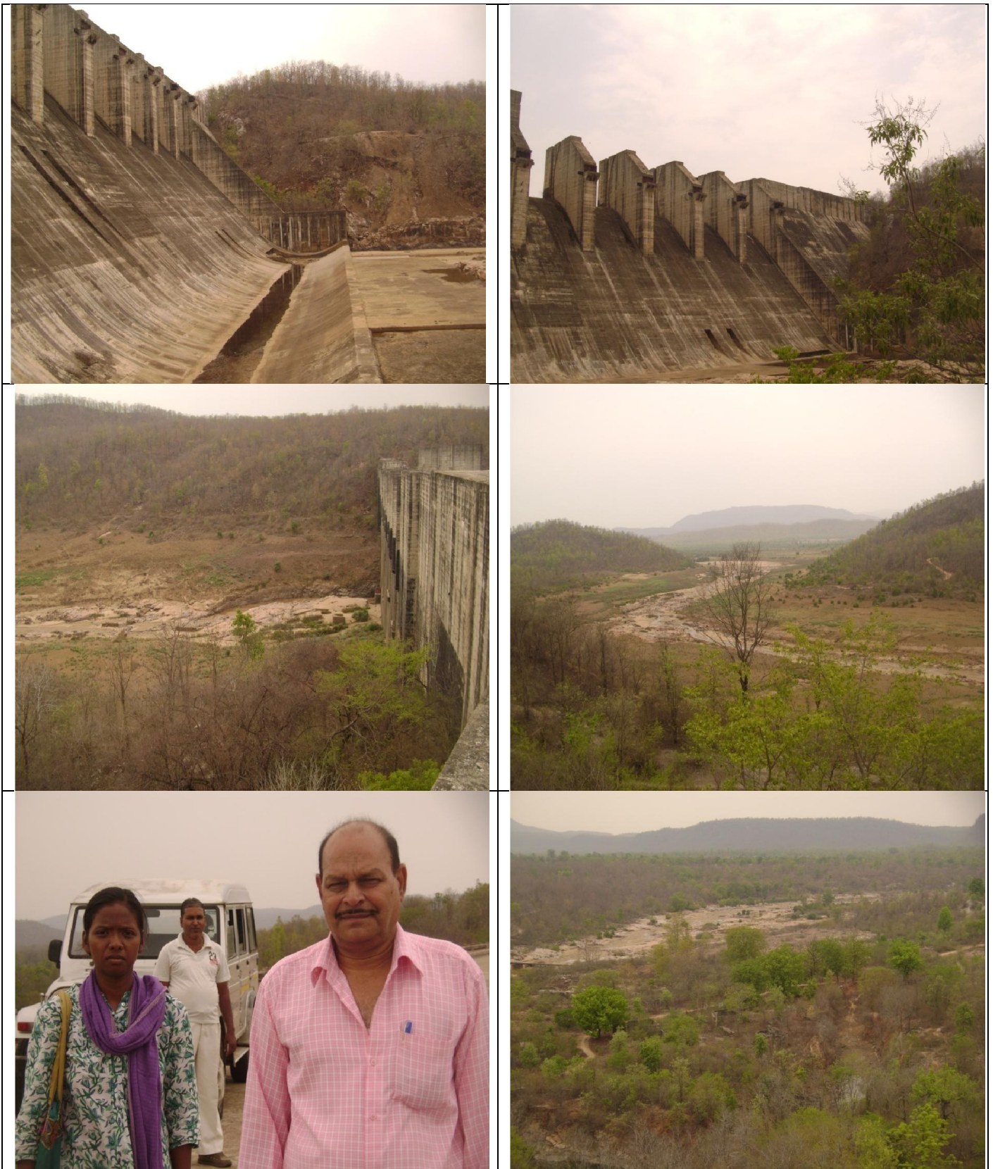
Figure 2: Mandal Dam Site Photograph-2
