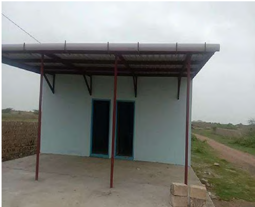
Renovation work carried out at Police Chowki in Kuranga Village, Dwarka
