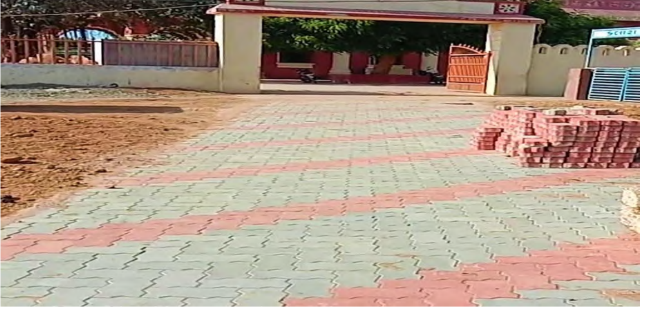
Laying of Paver Blocks at Nageshwar Temple, Dwarka
