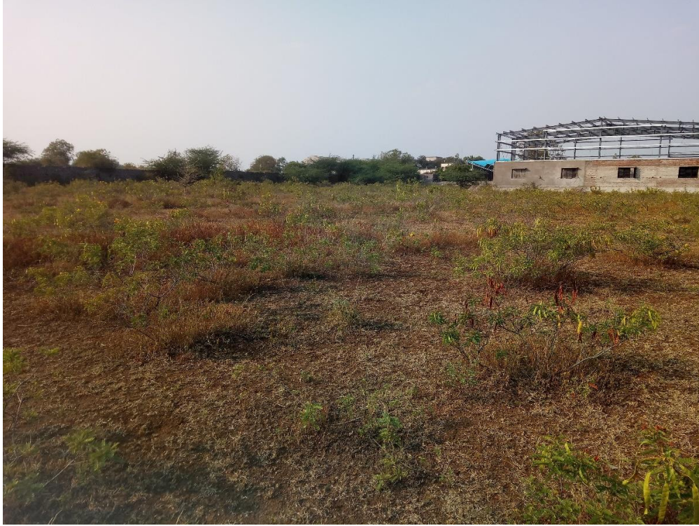
Figure No. 3 : Existing Site Photograph taken from North corner of the plot
