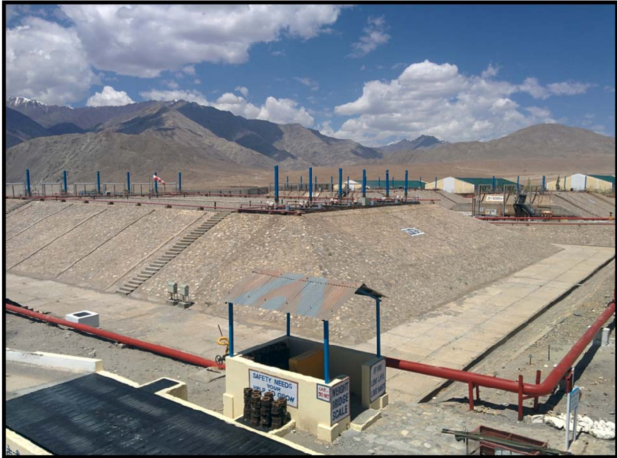
-Representative Picture from LEH LPG Bottling Plant
