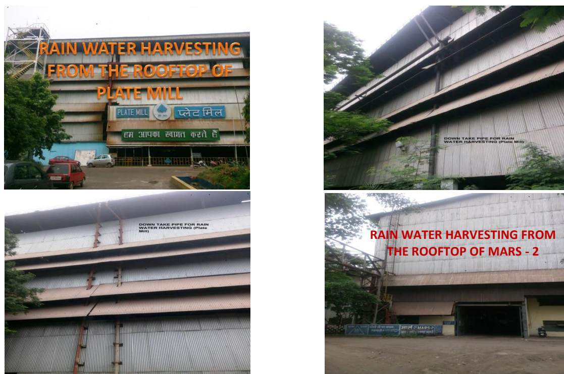
Fig 3.1: Roof Rainwater Harvesting Schemes Implemented Inside Plant
