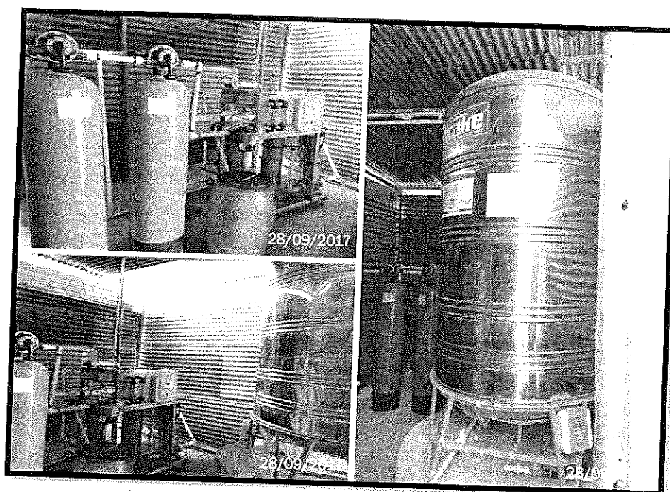
Fig. 4. RO-Plant in the labour camp.
