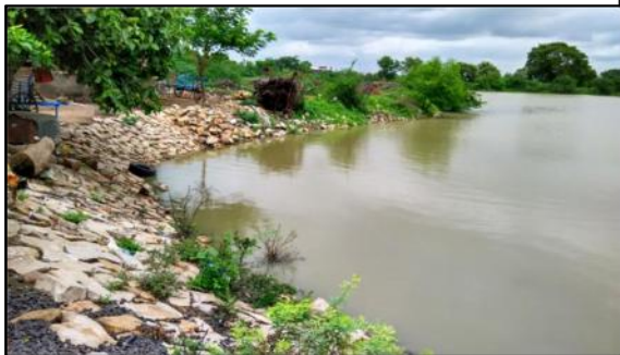
21. At Brahmani Village – Stone pitching and development of bund with pathway cement benches etc. of pond
