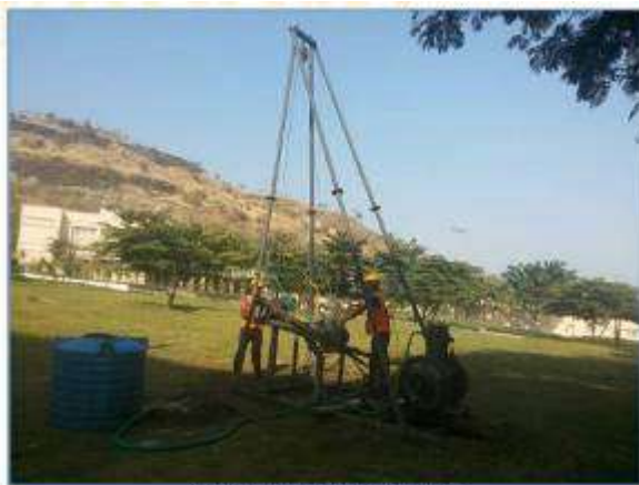
Borehole drilling in progress
