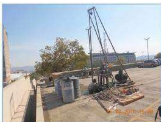
Borehole drilling in progress
