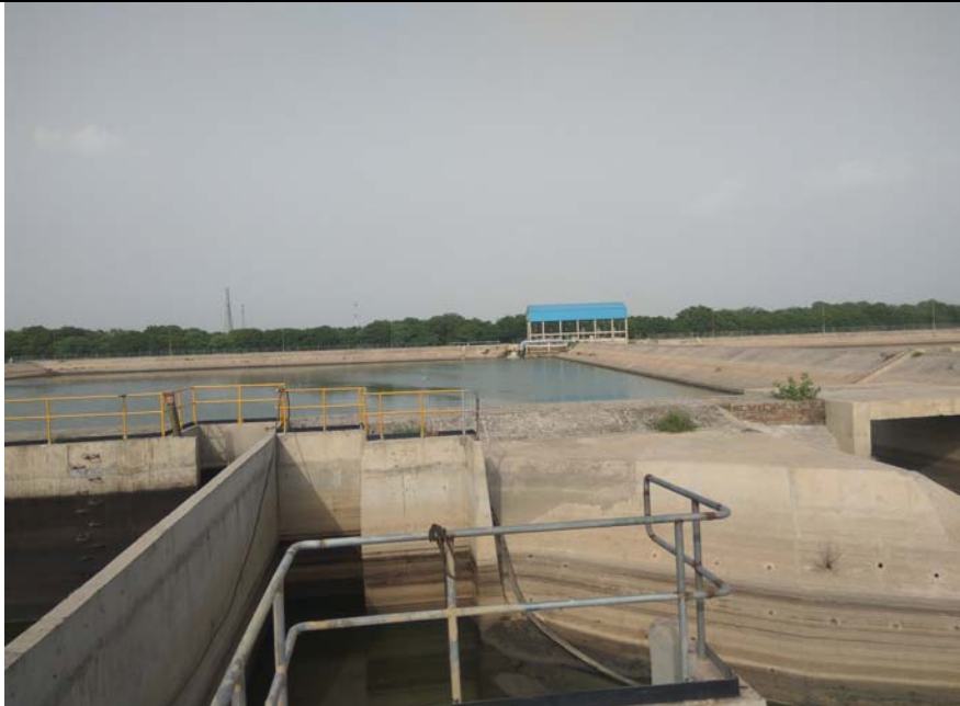
Photo 3: Showing status of storage of storm water pond having capacity of 172981 m 3
