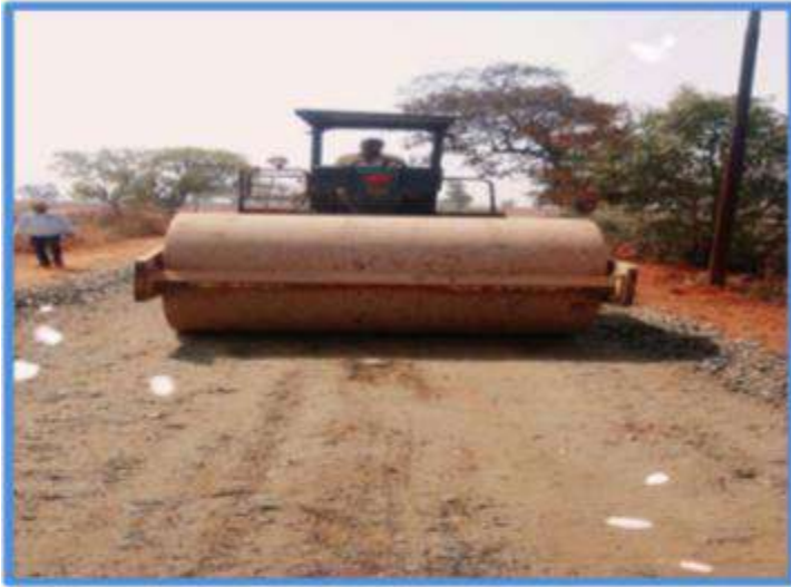
During WMM laying Work
