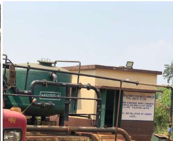
Multiple Pressure Sand Filter
