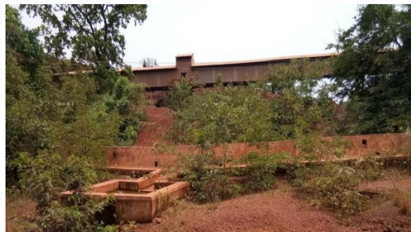
Retaining wall with garland drains & settling pit at Dump – 3 near DH - 5
