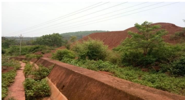
Retaining wall with garland drains & settling pit at Dump – 3 near DH - 5
