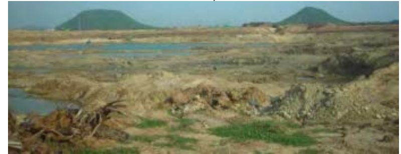
Figure 1.4 : View New Water Reservoir Site on 23-07-18 from approx. 17°40'41.8"N, 83°10'05.0"E
