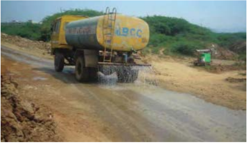
Figure 11.15 : Water Sprinkling on Road Between New Reservoir Site and Dump Site
