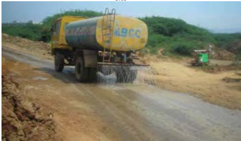
Figure 1.15 : Water Sprinkling on Road Between New Reservoir Site and Dump Site
