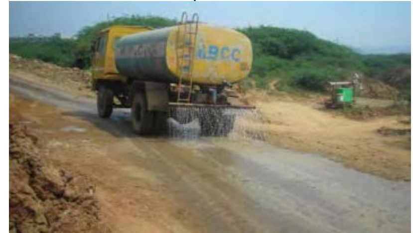
Figure 1.16 : Water Sprinkling on Road Between New Reservoir Site and Dump Site
