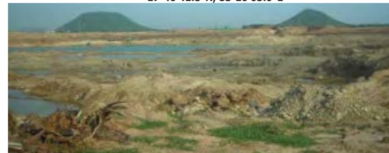
Figure 1.2 : View New Water Reservoir Site on 23-07-18 from approx. 17°40'41.8"N, 83°10'05.0"E
