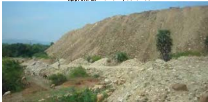
Figure 11.8 : Excavated Material from New Reservoir Dumped Externally at approx. 17°40'25"N, 83°07'33"E
