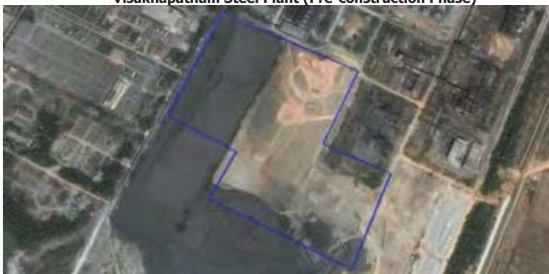
Figure 11.16 : Google Earth Image of 21st March, 2014 of Site of COB-5 inside Visakhapatnam Steel Plant (Pre-construction Phase)
