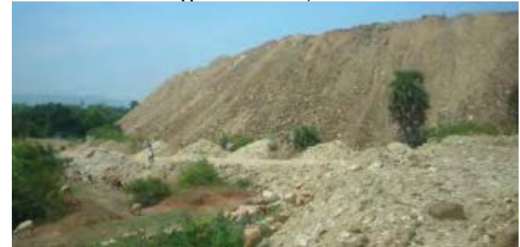
Figure 1.9 : Excavated Material from New Reservoir Dumped Externally at approx. 17°40'25"N, 83°07'33"E
