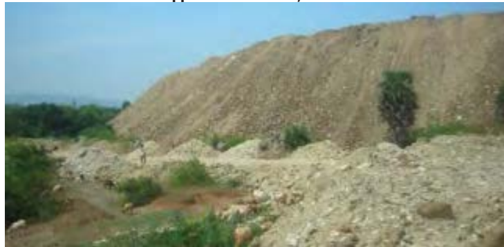
Figure 1.8 : Excavated Material from New Reservoir Dumped Externally at approx. 17°40'25"N, 83°07'33"E
